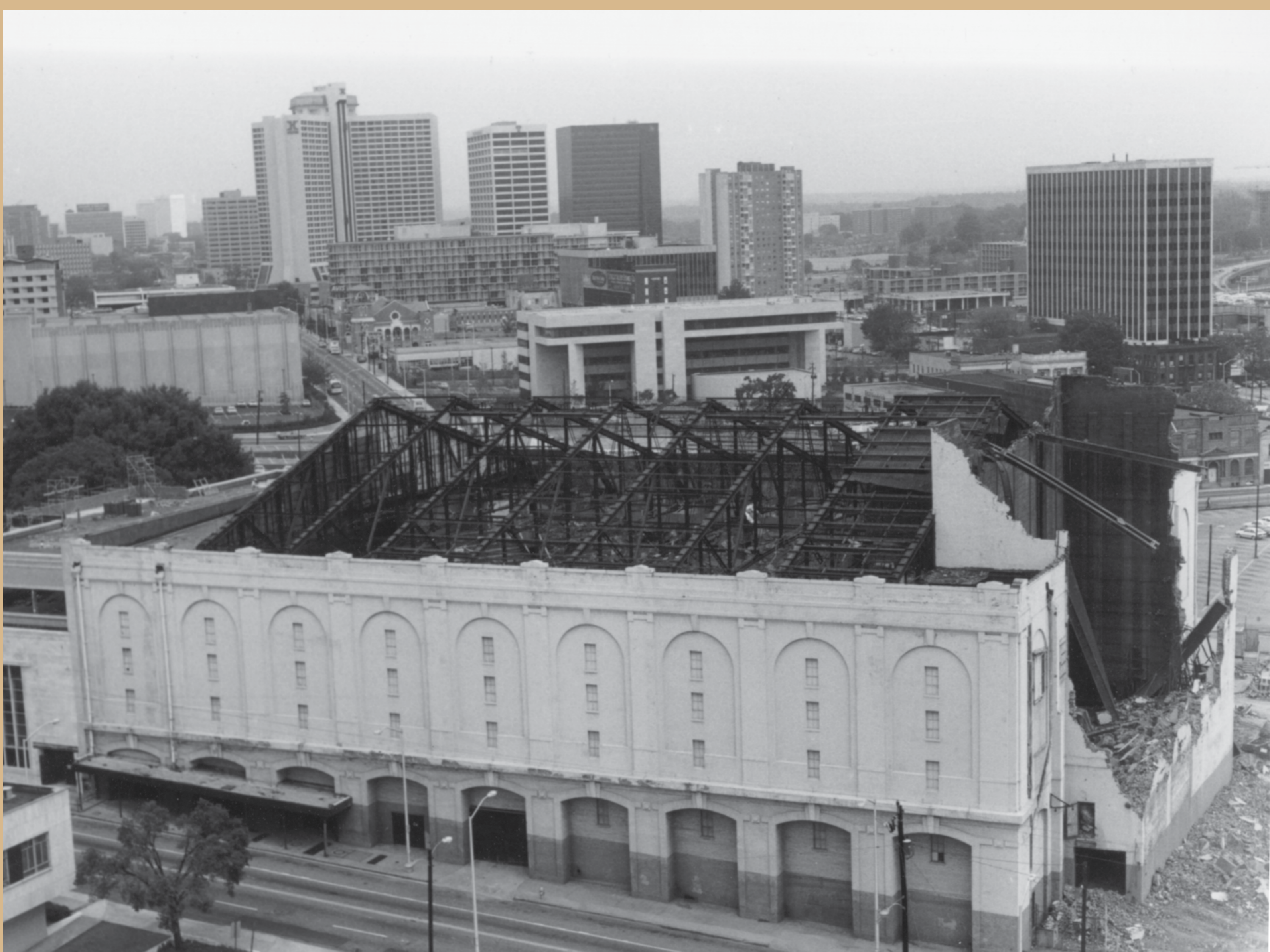
Demolition of the Auditorium, 1981
