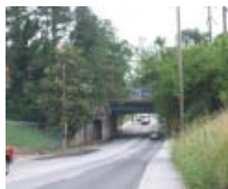
Northside Drive and 16th Street Bridge Underpass
