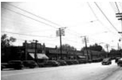
Peachtree adjacent to Peachtree Creek Bridge, 1952
