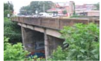
Peachtree Road overpass at CSX rail line
