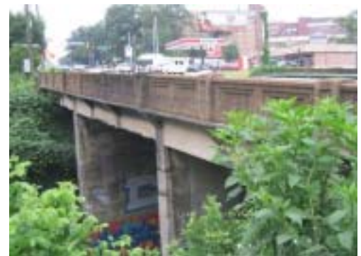
Peachtree Road Overpass
