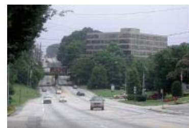
Northside Drive Overpass
