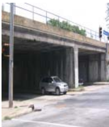
Ralph David Abernathy Overpass
