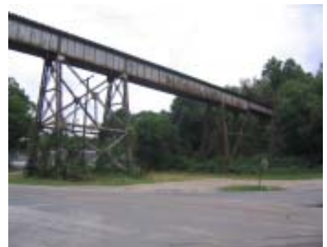
North Avenue Overpass
