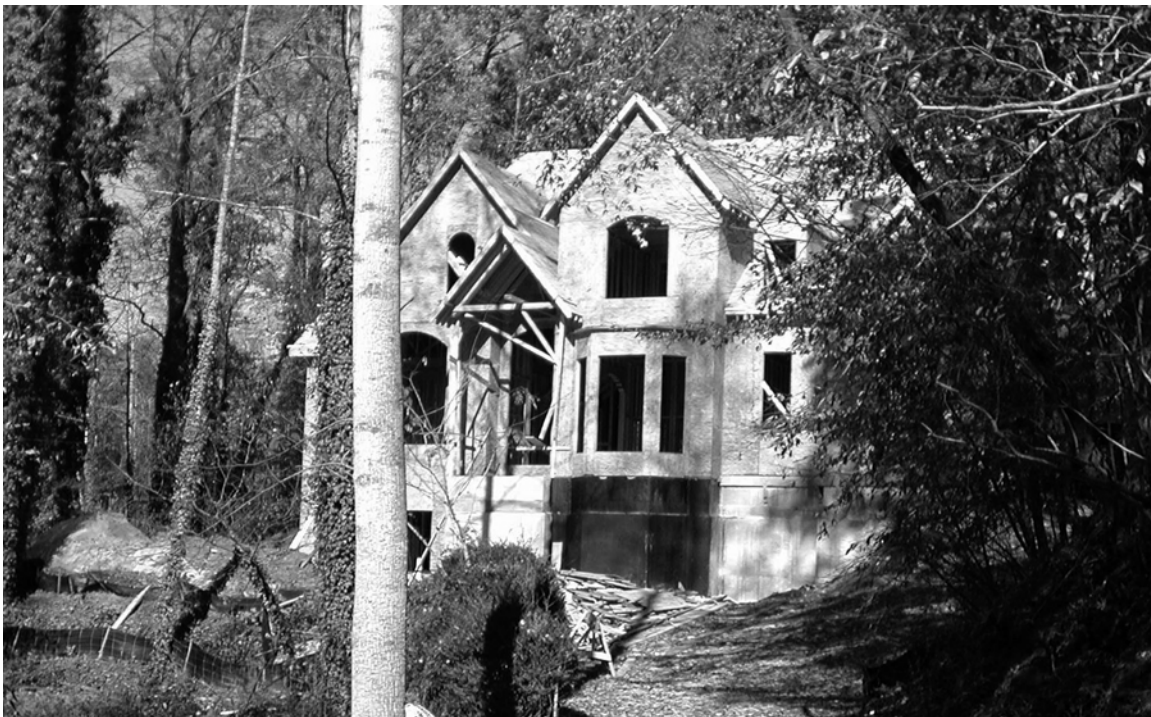
Figure 10. New infill home being built near Peachtree-Dunwoody Rd., 2004 Source: Author
