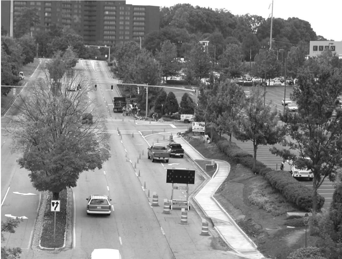
Figure 20. Hammond Drive sidewalk improvements near Ashford-Dunwoody and Perimeter Mall, 2004 Source: Author
