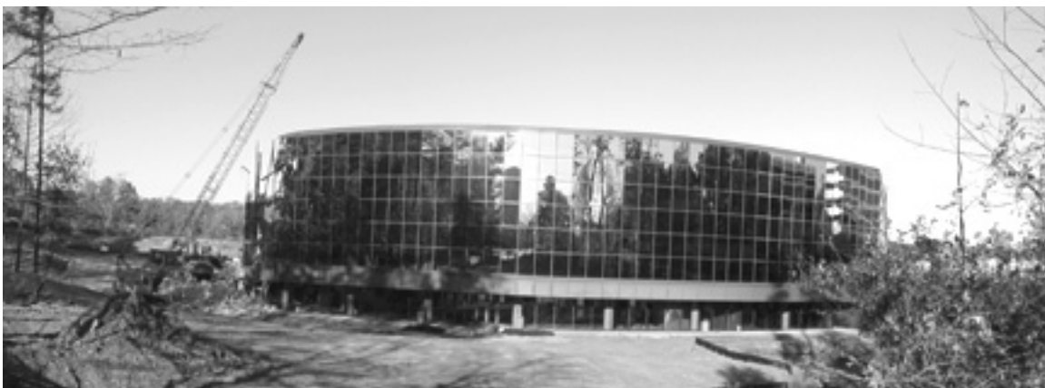
Figure 12. The removal of a vacant office building, 2004 Source: Author
