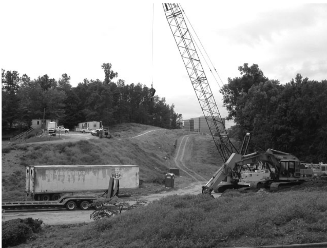
Figure 19. Northern construction site of “fly-over” bridge at I-285, 2005 Source: Author
