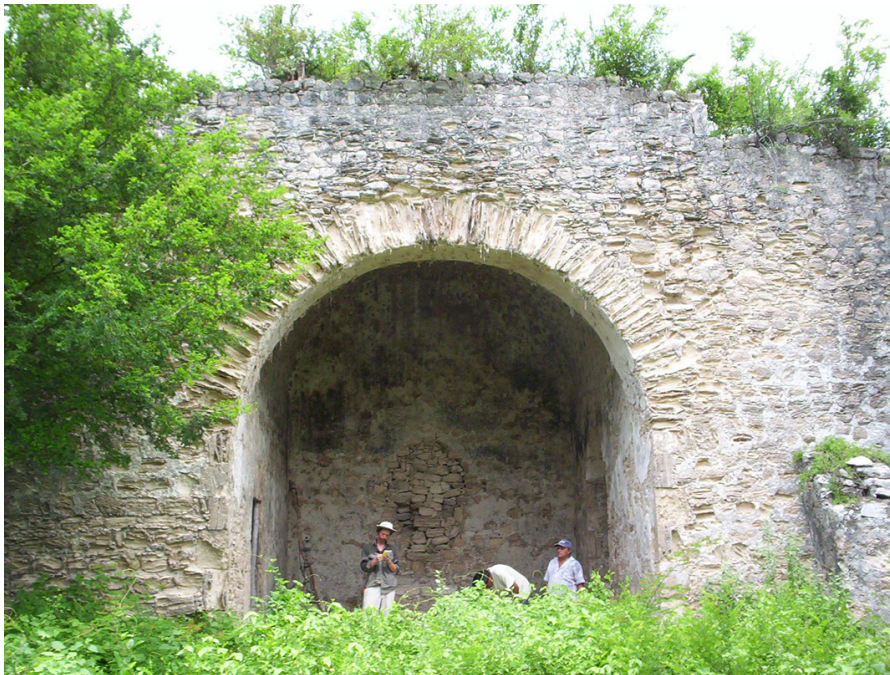
Figure A.24: The interior portion of the church.
