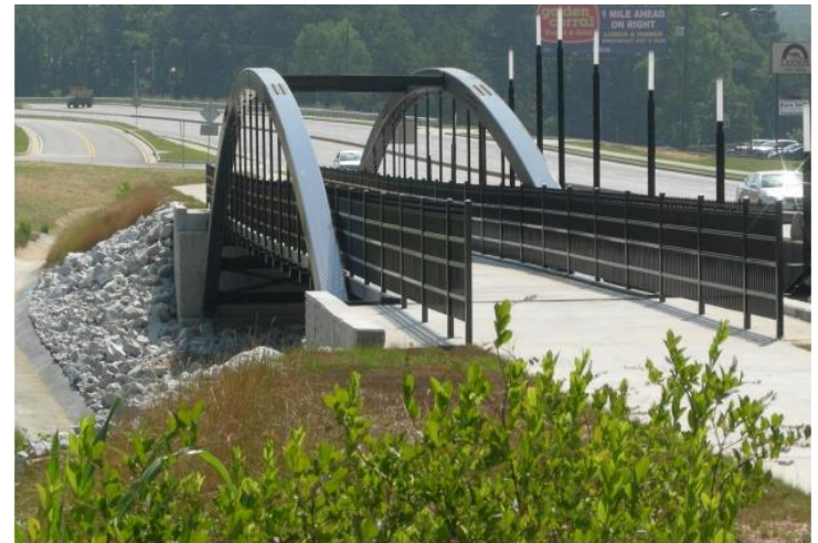
Yellow River Pedestrian Bridge
