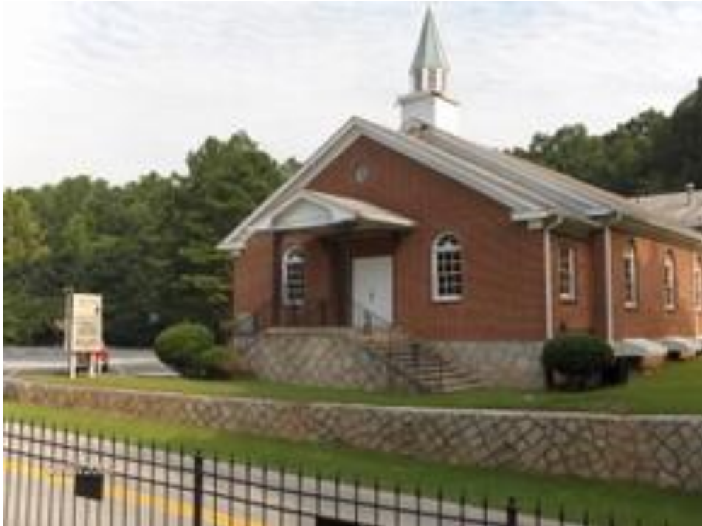
6910 South Goddard Road Philadelphia Baptist Church (ca. 1955) Granite is used in the steps, foundation and retaining wall.
