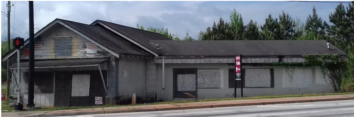
Commercial building at corner of Browns Mill Road and Klondike Road. Example of a Cross-Gabled Roof.
