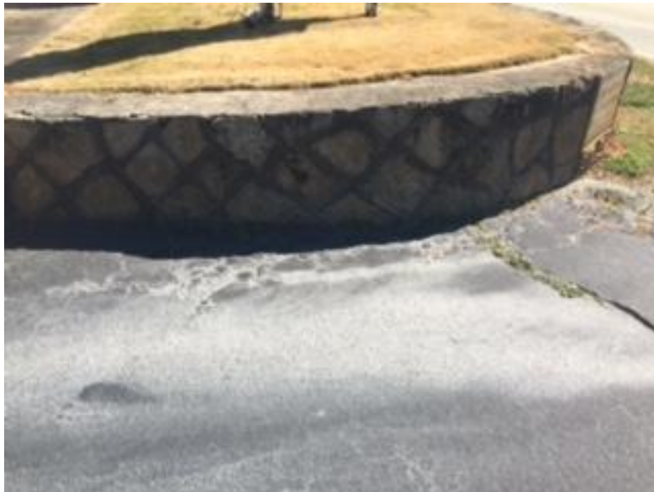
Example of granite retaining wall.
