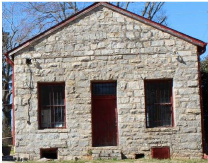
The “Oak Grove Junction Convenience Store,” located at the crossroads of Klondike Road and South Goddard Road. Example of a Front-Gabled Roof.
