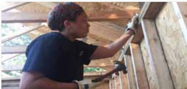
New homeowner Tori Hitchcock and her father were at the build every week!
