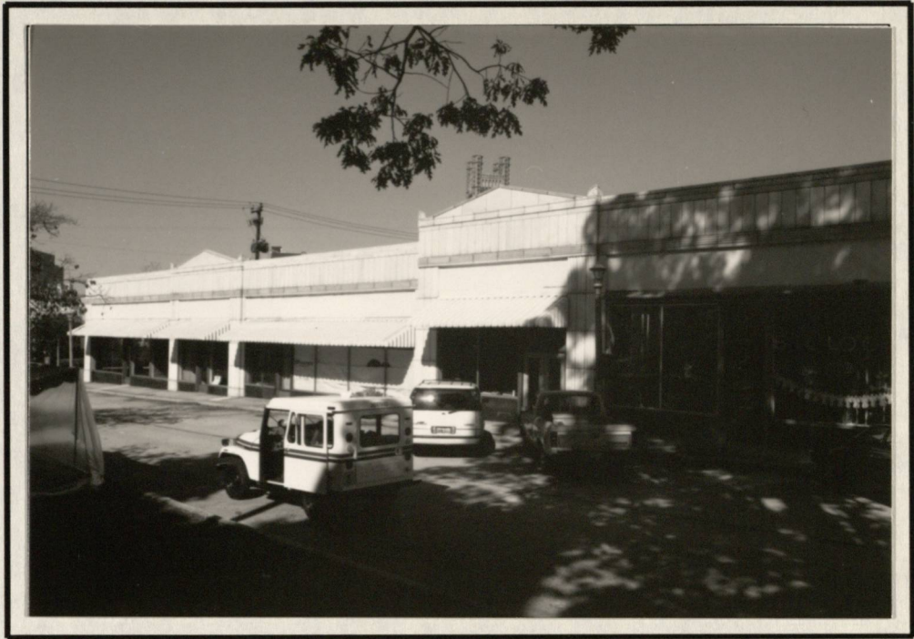
NORTH RHODES CENTER - SOUTH ELEVATION (FROM LEFT) STORE #10, #9, #8,#7, AND #6
