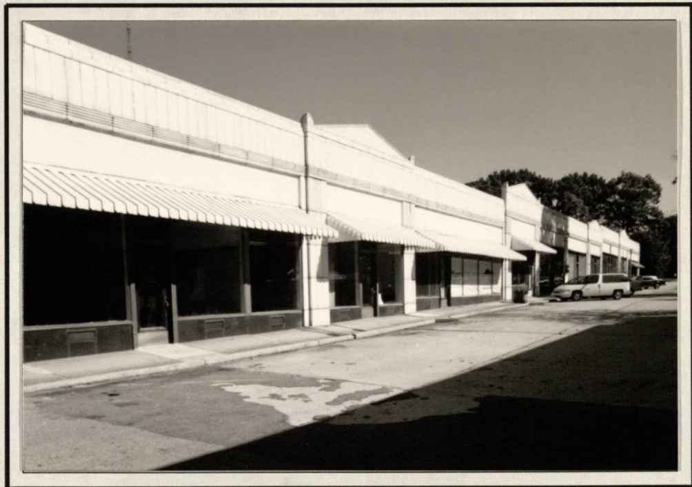
NORTH RHODES CENTER - SOUTH ELEVATION VIEW LOOKING FROM SOUTHWEST
