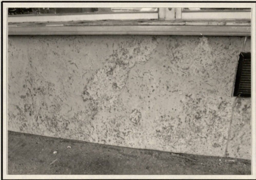
WEST RHODES CENTER - WEST ELEVATION MARBLE DETAIL - RIGHT OF DOORS
