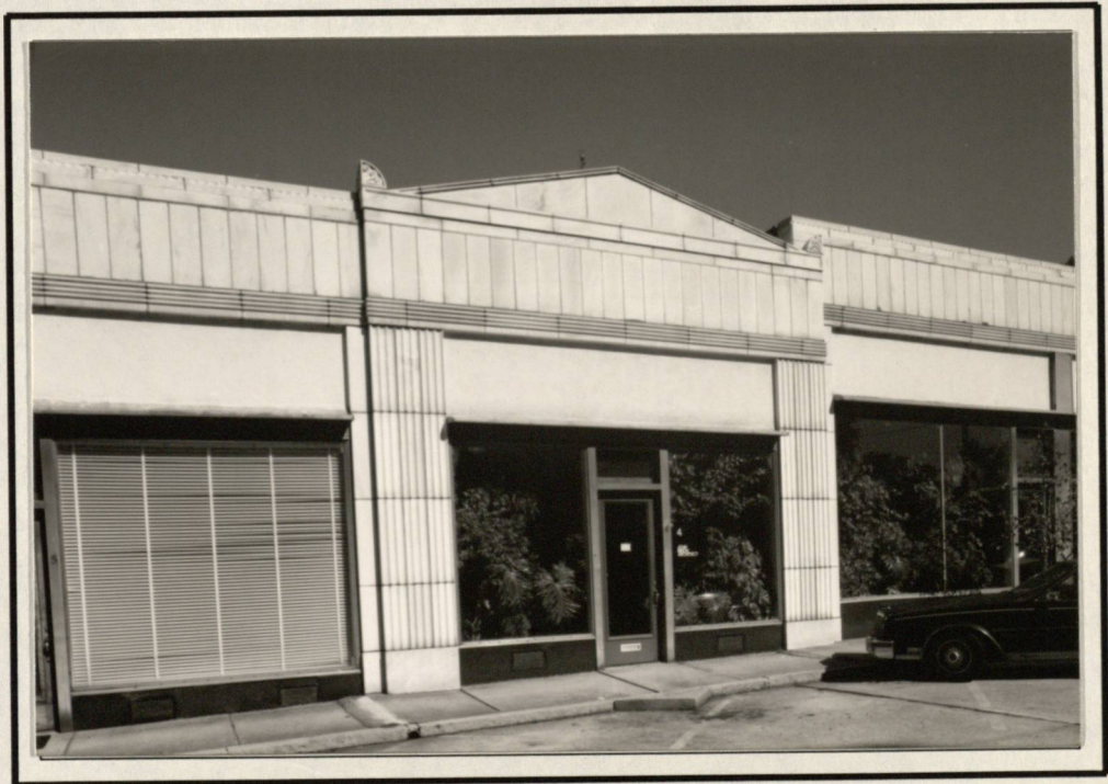
NORTH RHODES CENTER - SOUTH ELEVATION (FROM LEFT) STORE #5, #4 AND #3
