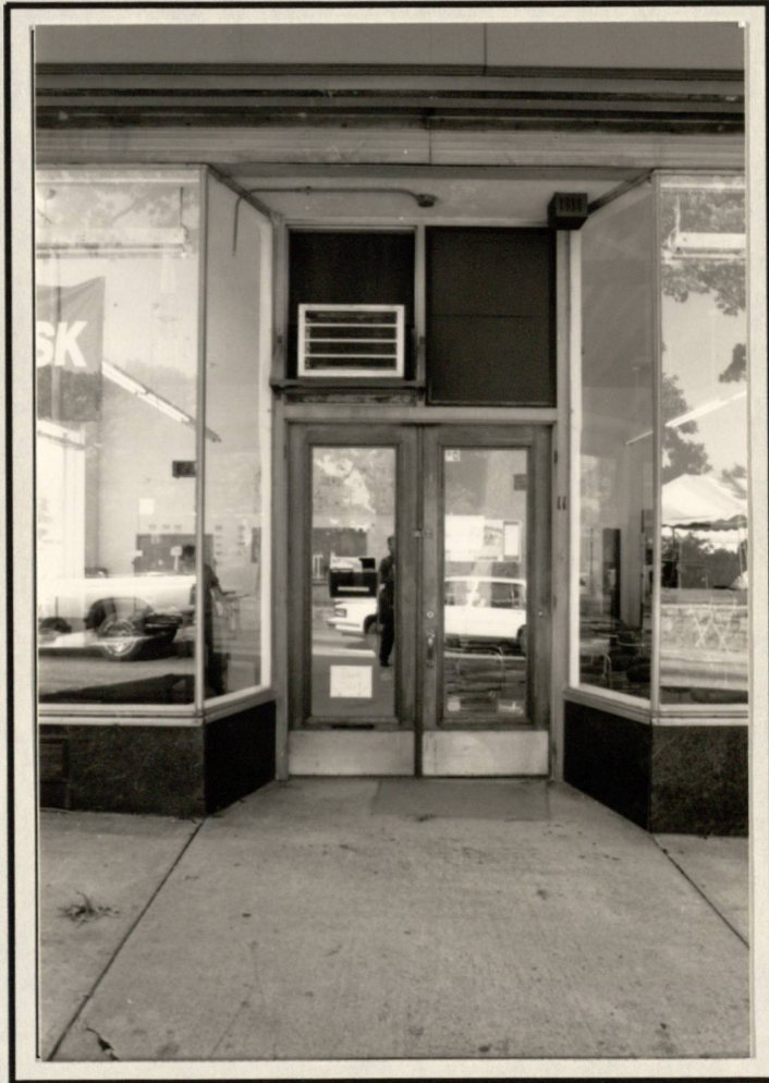
SOUTH RHODES CENTER - NORTH ELEVATION STORE #11 ORIGINAL ENTRANCE DOORS
