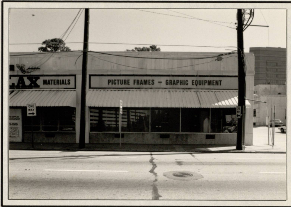
WEST RHODES CENTER - WEST ELEVATION RIGHT SIDE (FACING BUILDING)
