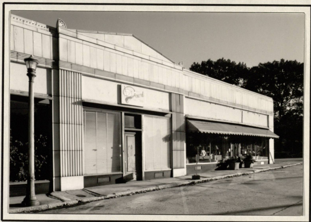
NORTH RHODES CENTER - SOUTH ELEVATION (FROM LEFT) STORE #2 AND #1
