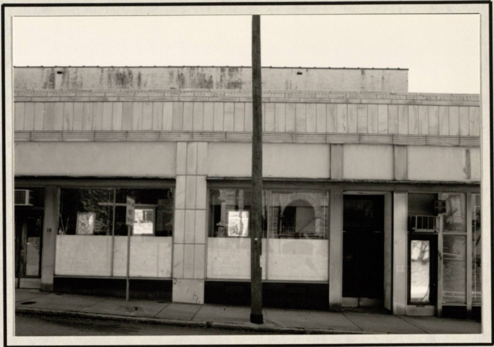
SOUTH RHODES CENTER - NORTH ELEVATION (FROM LEFT) STORE #16, THEATER EXIT & #17
