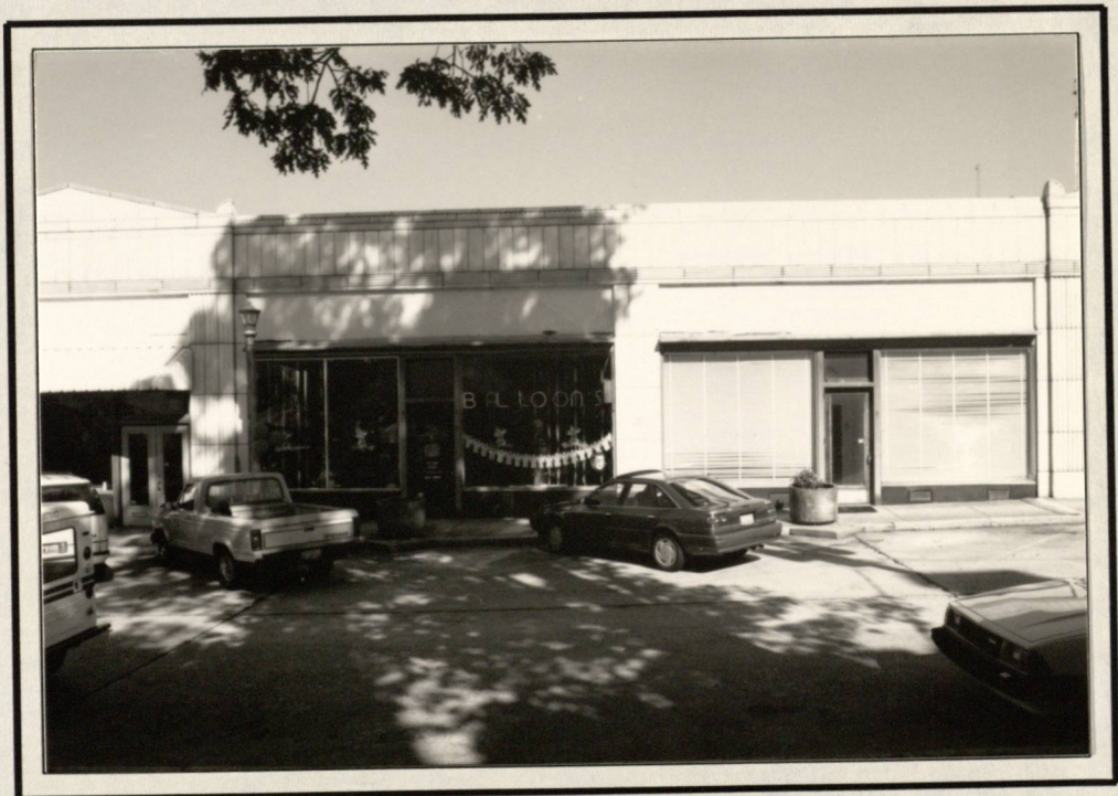
NORTH RHODES CENTER - SOUTH ELEVATION (FROM LEFT) STORE #1, #4 AND #5
