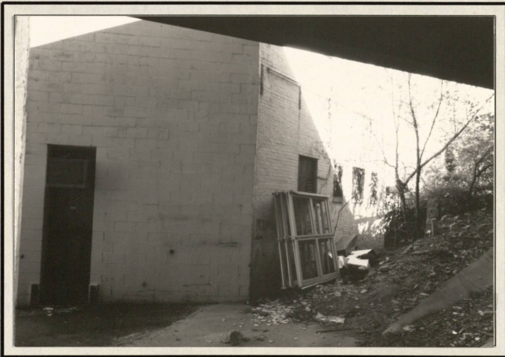
SOUTH RHODES CENTER - LOOKING EAST NORTHEAST
