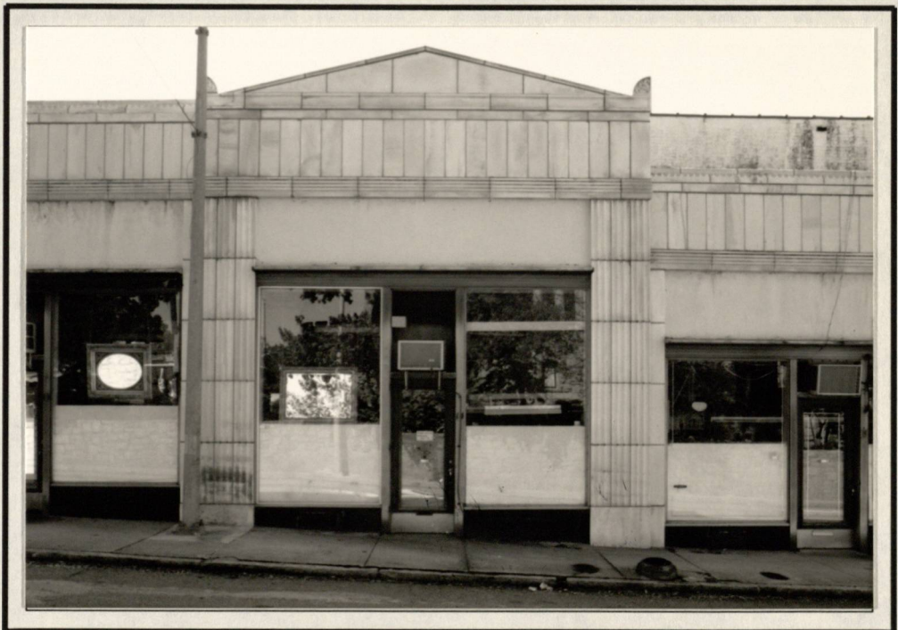
SOUTH RHODES CENTER - NORTH ELEVATION (FROM LEFT) STORES #13, #14, & #15
