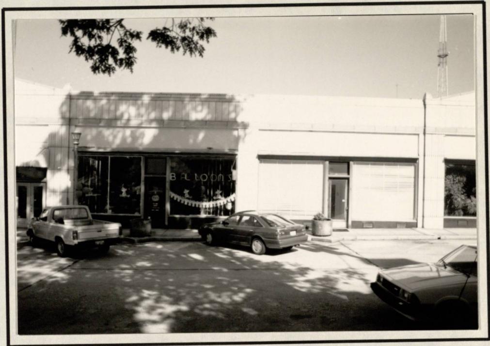
NORTH RHODES CENTER - SOUTH ELEVATION (FROM LEFT) STORE #4 AND #5
