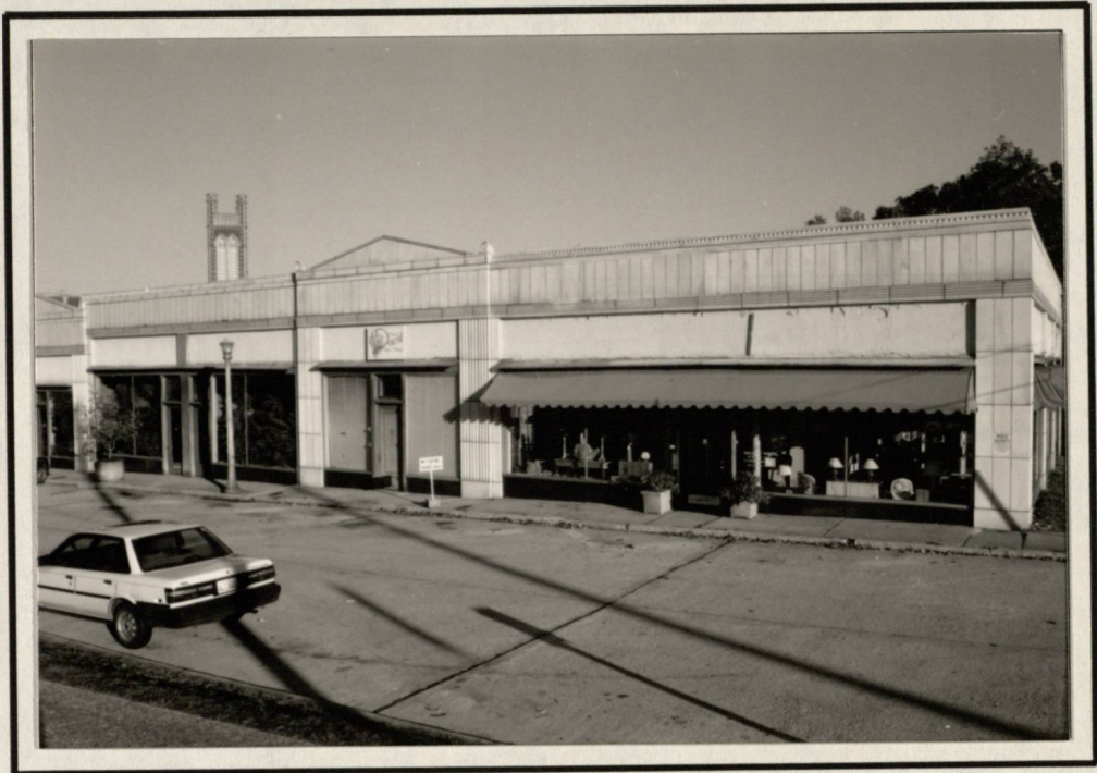
NORTH RHODES CENTER - SOUTH ELEVATION (FROM LEFT) STORE #3, #3A, #2 AND #1
