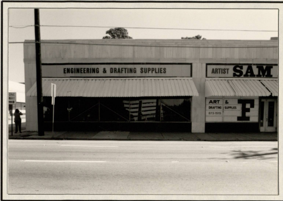
WEST RHODES CENTER - WEST ELEVATION LEFT SIDE (FACING BUILDING)
