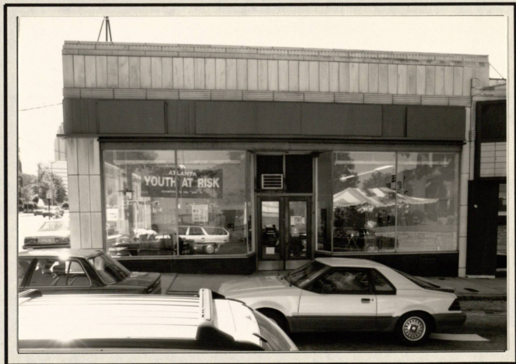
SOUTH RHODES CENTER - NORTH ELEVATION STORE #11
