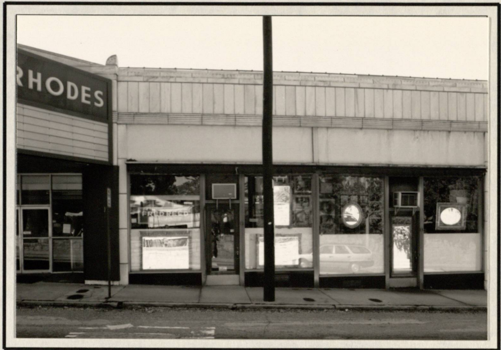
SOUTH RHODES CENTER - NORTH ELEVATION (FROM LEFT) THEATER, STORE #12, AND #13
