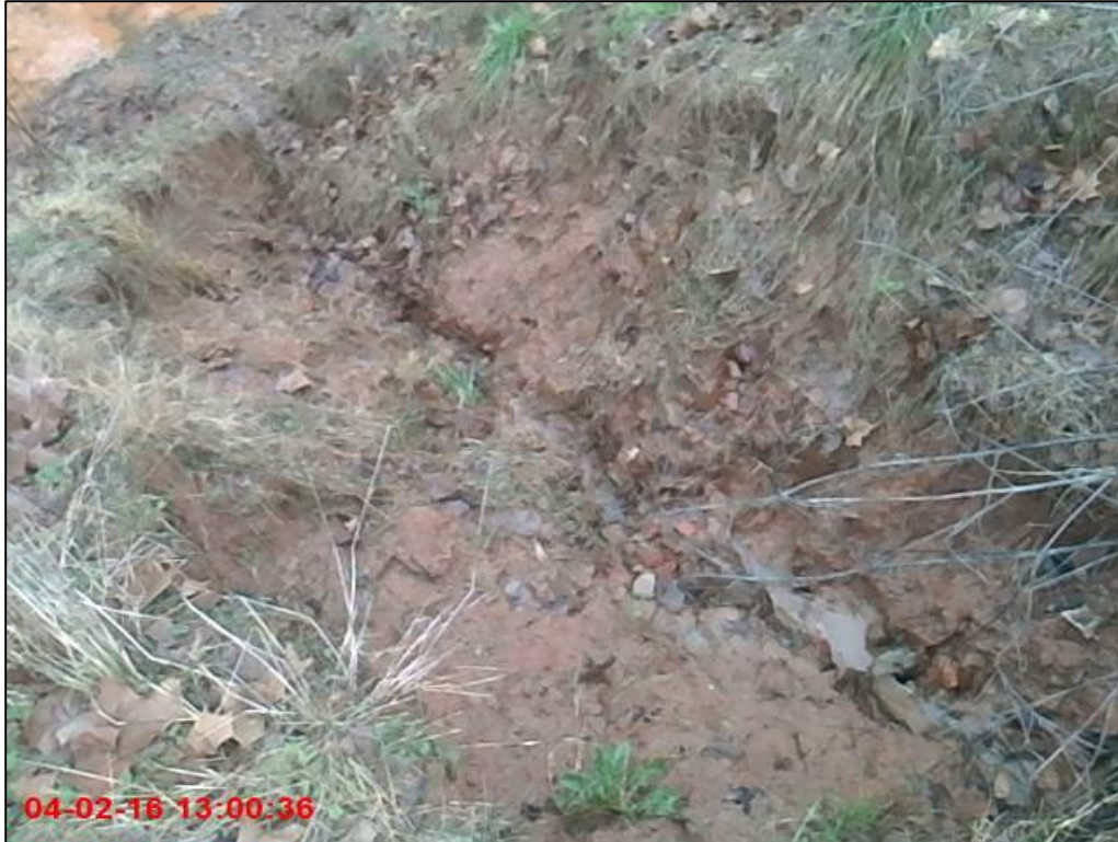
Figure 10: Gully in sink area
