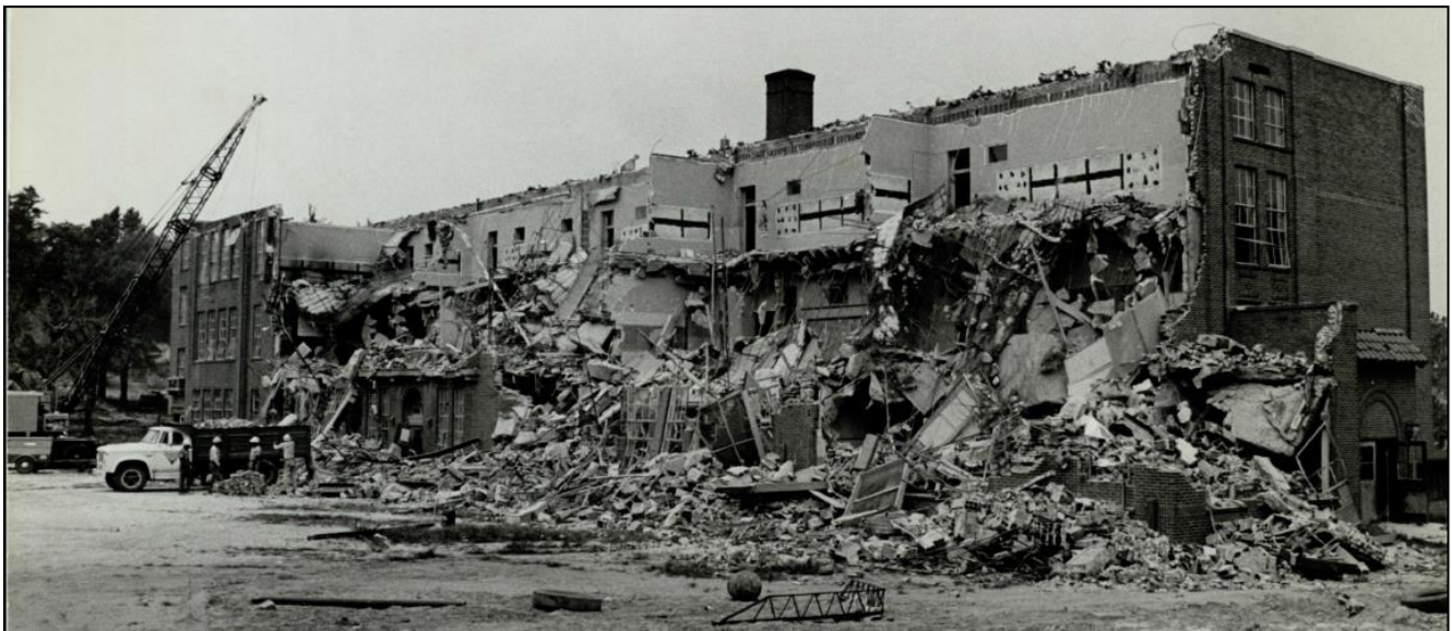
Figure 3: Demolition of C.W. Hill Elementary School (GSU Special Collections)
