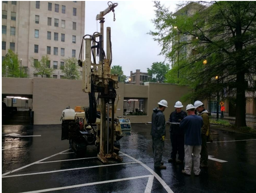
Figure 2.3 At the SB02 location, the drilling operation was unsuccessful
