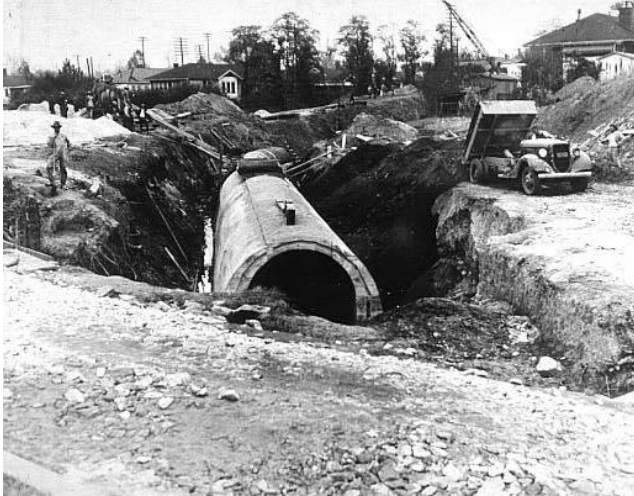
Figure 1.2 Photograph of construction on Atlanta Connally Sewer (WPA, 1936).
