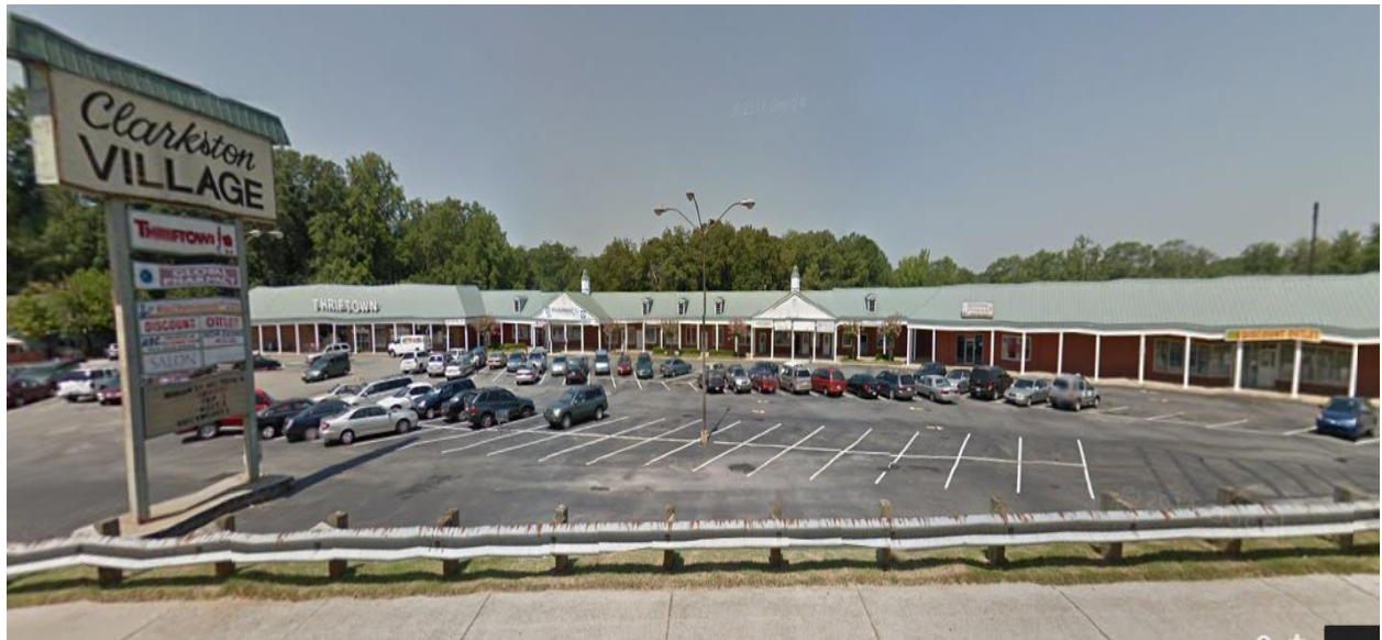
Figure 3.6.3.1 Clarkston Village Shopping Center
